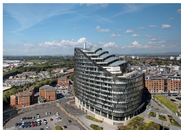
Figura 76 – One Angel Square, Manchester (GBR) Fonte: 3D Reid, 2013
