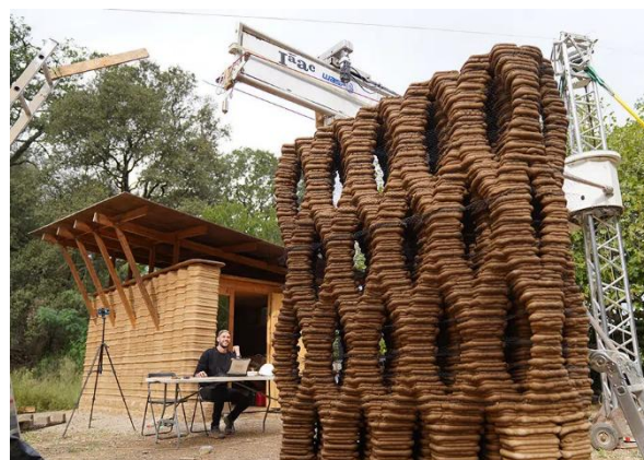
Figura 111 – Hope Village Community Building: Protótipo, Forest Campus do IAAC, Catalunha (ESP). Fonte: IAAC, 2025.
