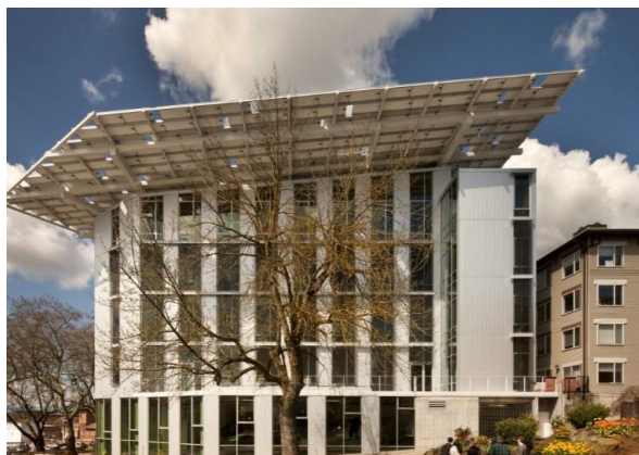
Figura 81 – The Bullitt Center, Seattle (EUA) Fonte: The Miller Hull Partnership, 2013
