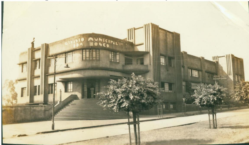
Figura 10: Fachada do Gymnasio Municipal Dom Bosco
