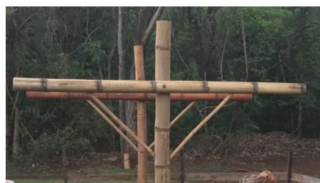
Diagonals fastened with screws.
