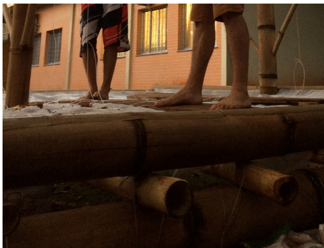
When climbing the table to perform any work step, use wooden planks to avoid deforming the chicken wire.
