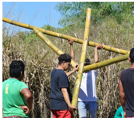
Diagonals fastened with threaded bars.
