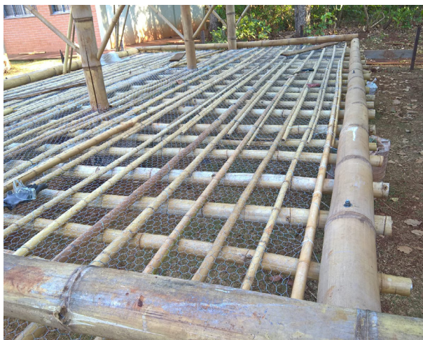
The wire has to cover the entire table, but the edges.
