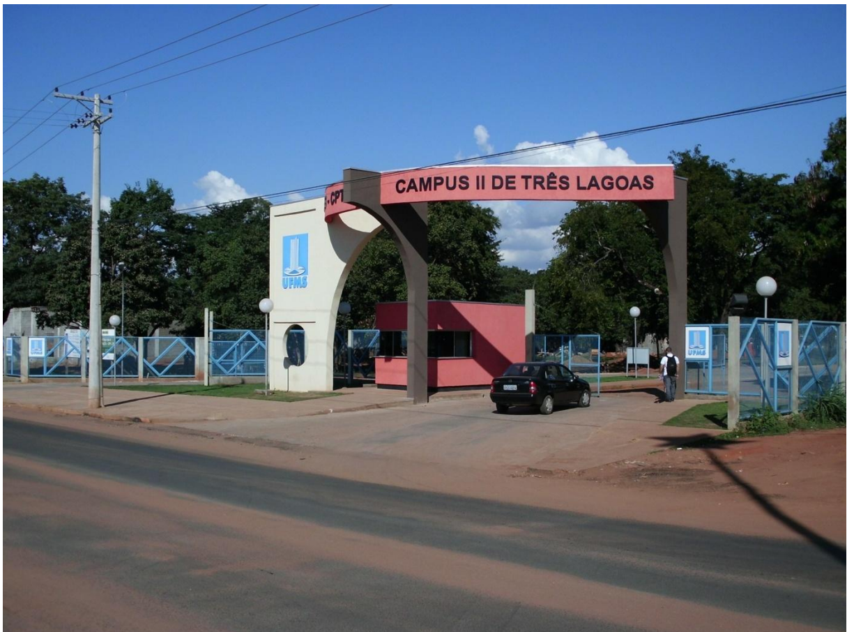
Figura 3.1 – Fachada principal do CPTL II
